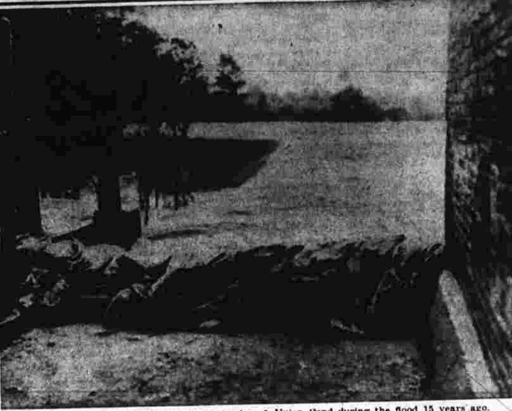
Sandbags were needed to contain the banks of Union Pond during the flood 15 years ago.
